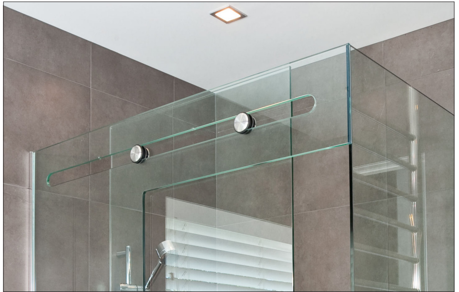
Figure 51 Edgework and Cut Outs in a Shower Screen Source: Viridian
