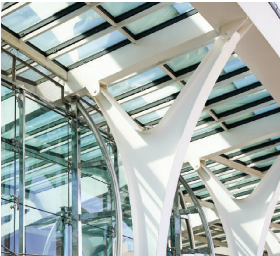
Figure 22 Sloped Overhead Glazing Source: Shutterstock
