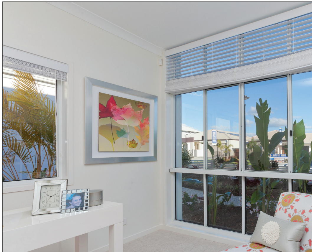
Figure 20 Low Level Glazing and Full Height Windows Source: G.James
